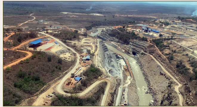
The dam construction site at Steigler's Gorge
